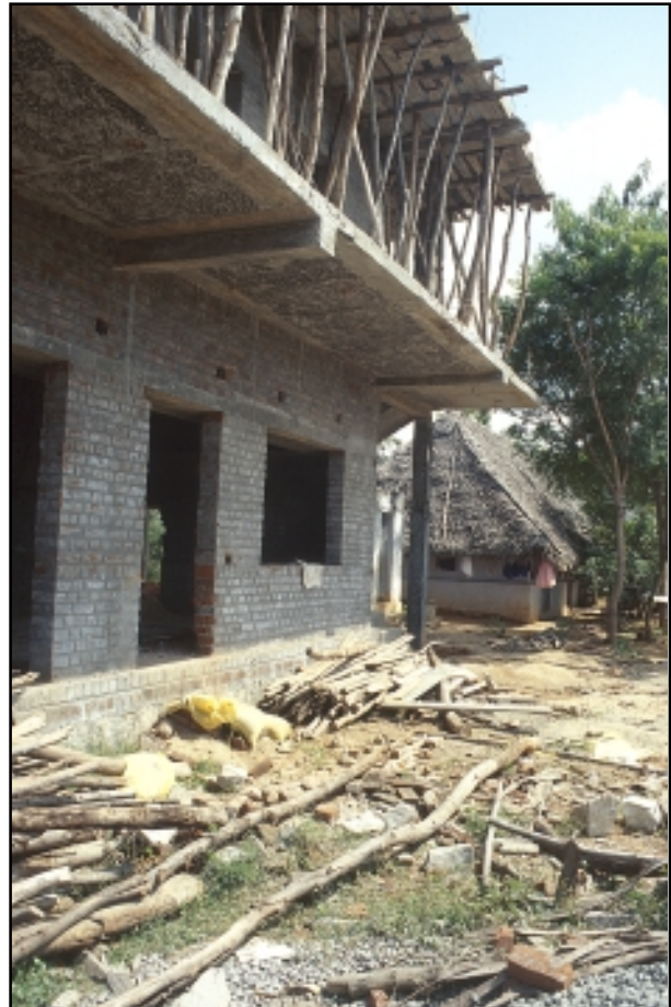
The new children's home under construction.
